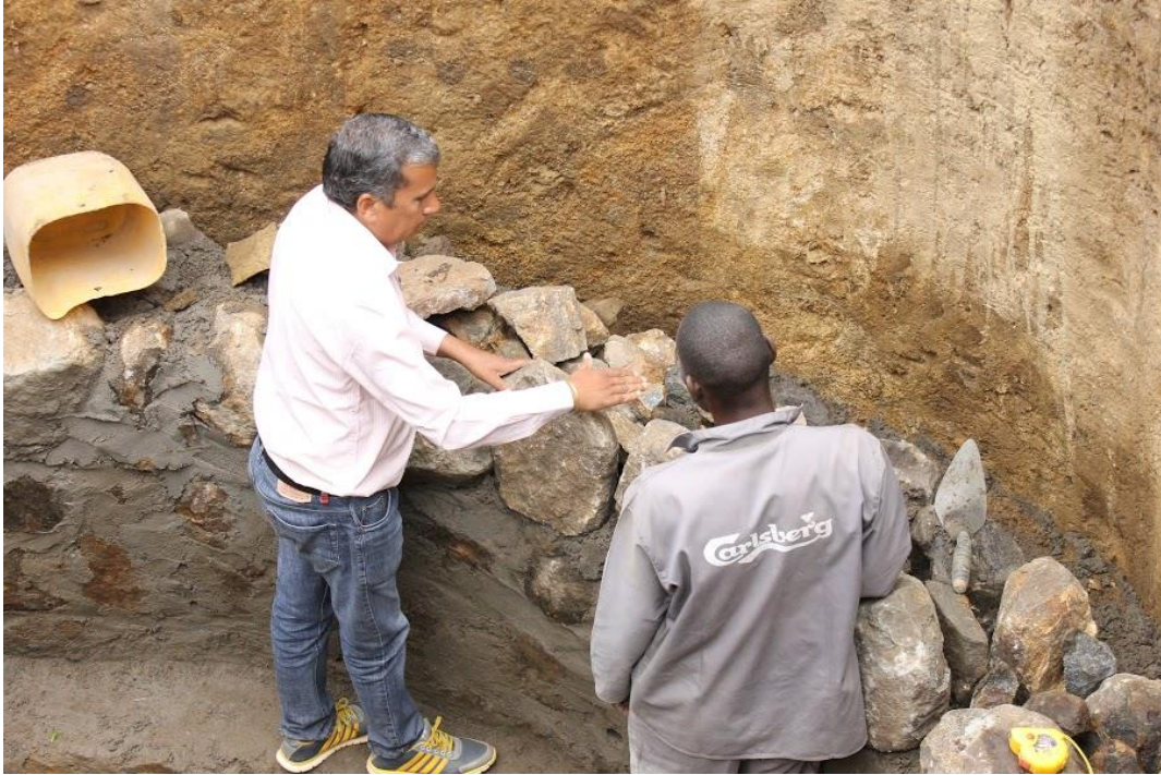
Laying the stone to form the interior structure of the well.
