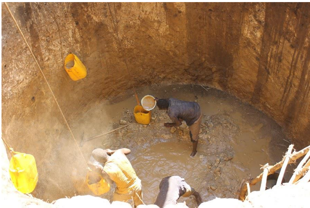
Excavation of soil to form the well.
